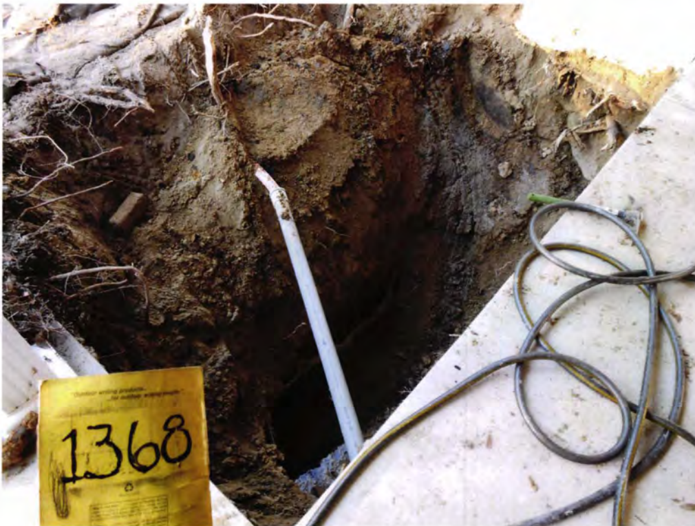
Picture 2: UST 1368Cardinal excavation.
